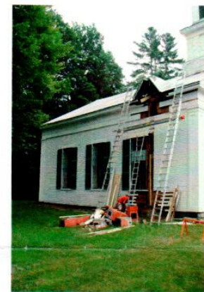
Removal of the cricket and repair surrounding damage.
